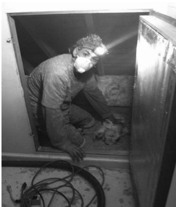
Installation work by Energía worker.
