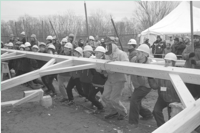
Construction starts at the new River Valley Co-op Market in Northampton, MA. The timbers in the photo were produced by the Massachusetts Woodlands Co-op in S. Deerfield, MA.
